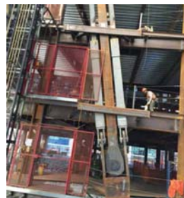
BRB(Buckling-restrained brace)とdamperを導入したmega-brace
