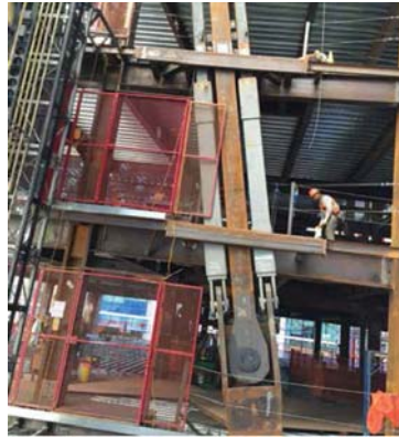
BRB(Buckling-restrained brace)とdamperを導入したmega-brace
