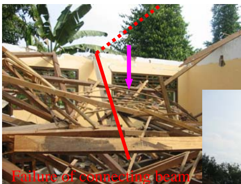
SD2 Putren, constructed in 2005
