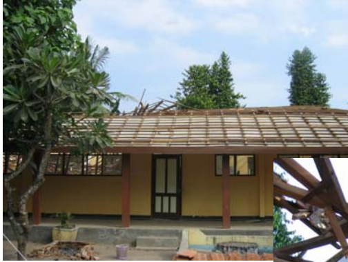
SD2 Putren, constructed in 2005
