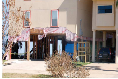
Breakaway walls beneath this building failed as intended under the flood forces of the 2008 Hurricane Ike.
