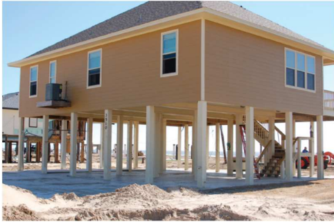
Breakaway walls beneath this building failed as intended under the flood forces of the 2008 Hurricane Ike.
