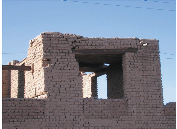
(b) Simple Masonry (Vulnerability class B).
